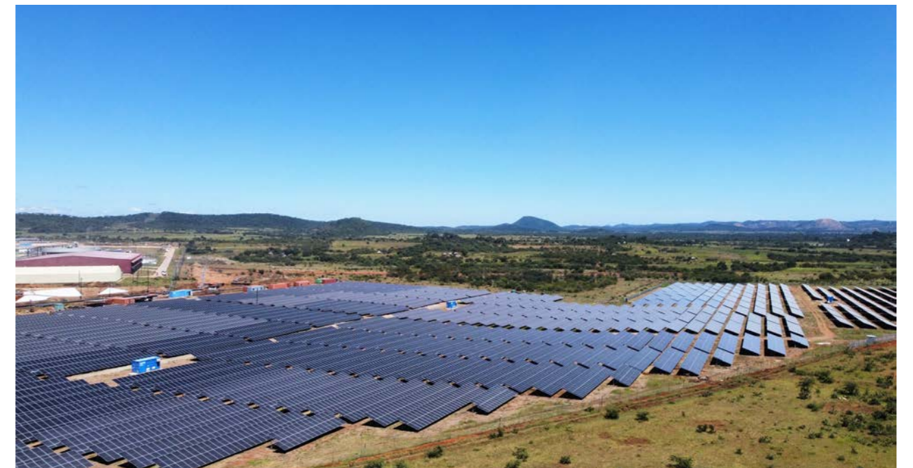
Operational commissioning of the Bikita Mine photovoltaic power plant
